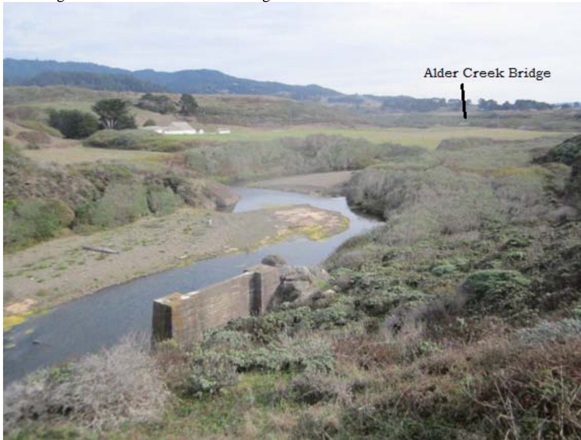
Photo 6. Same view as Photo 5 but from slightly further east; showing remains of old Alder Creek Bridge destroyed by fault rupture in 1906 earthquake.
