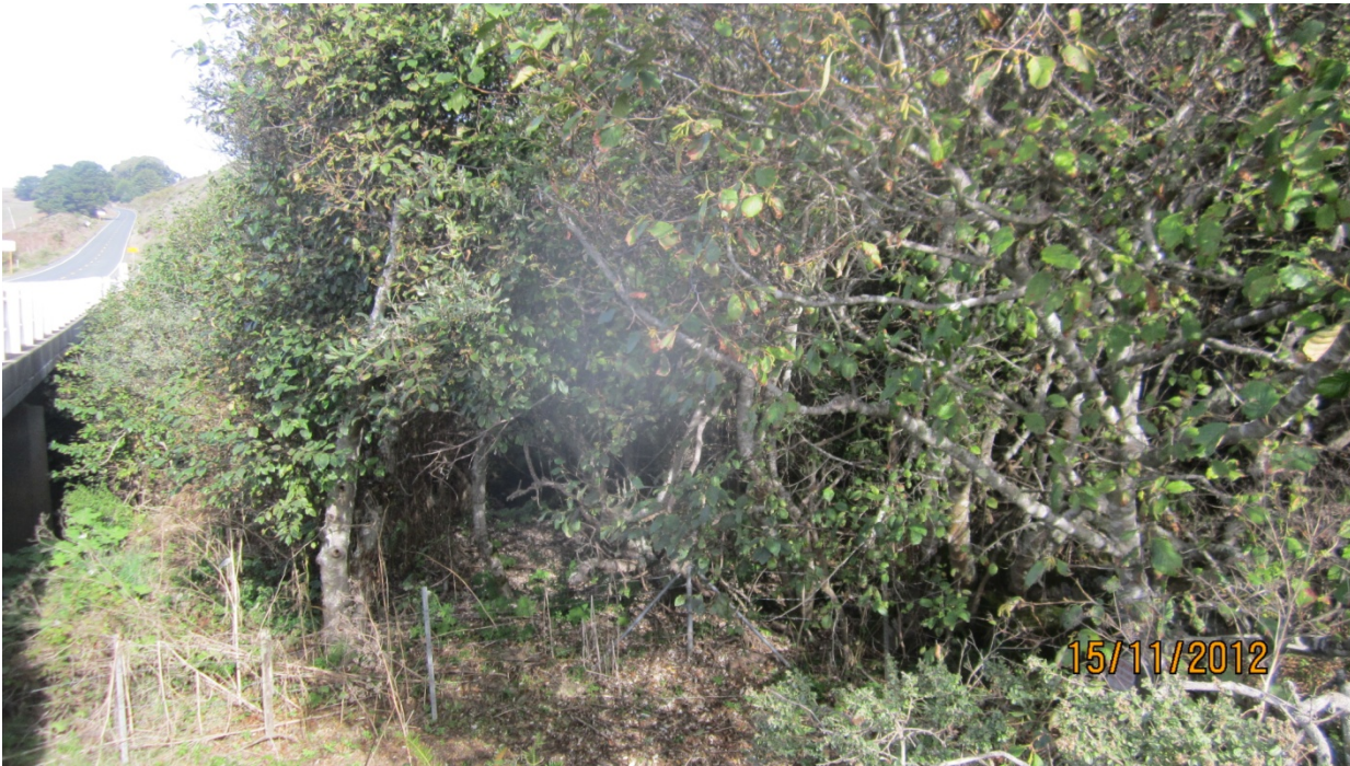
Photo 3. Looking southerly along Alder Creek Bridge.
