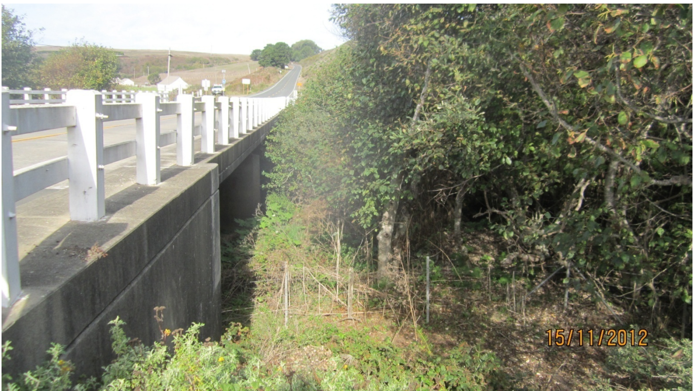
Photo 2. Looking northerly at Alder Creek Bridge.
