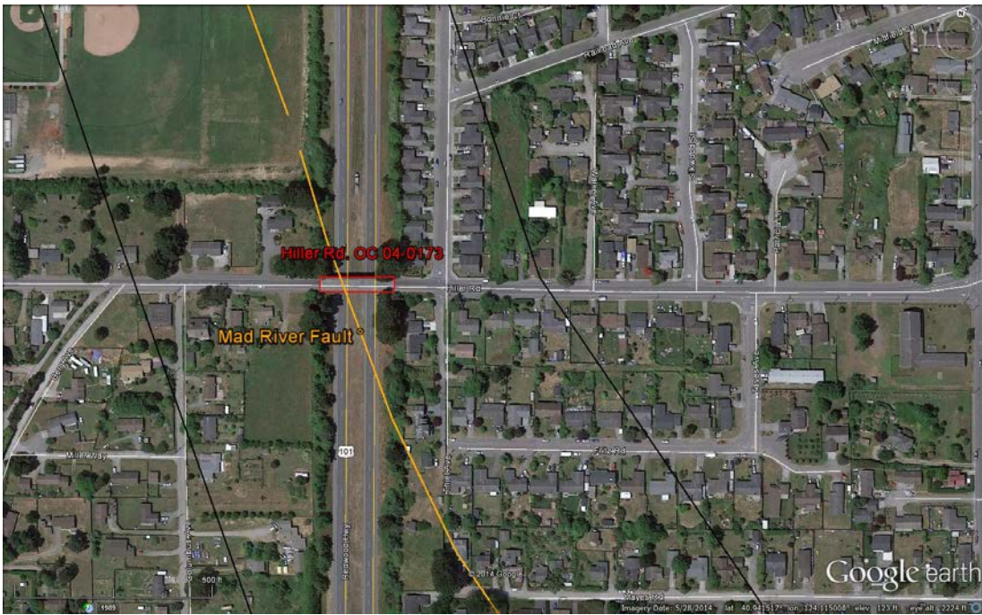
Figure 1. Hiller Road Overcrossing, with fault trace and EFZ boundaries (after USGS/Google Earth Faults, 2014).
